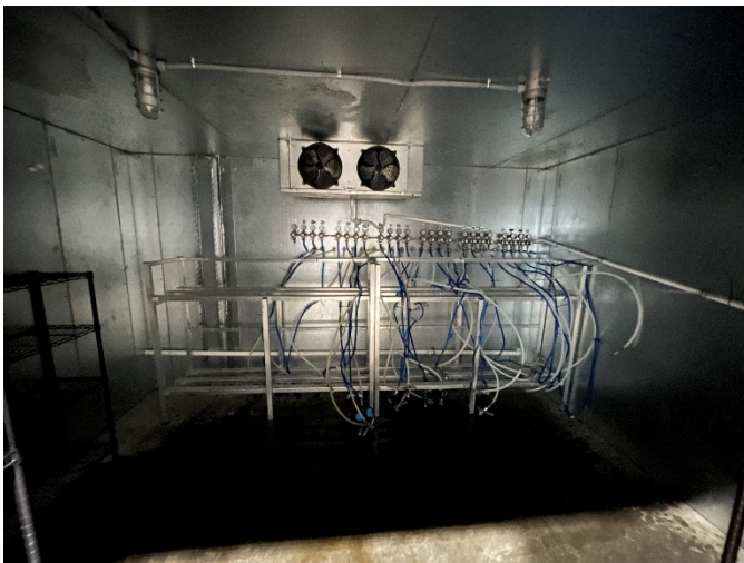
Walk-in Cooler With Tap Lines
