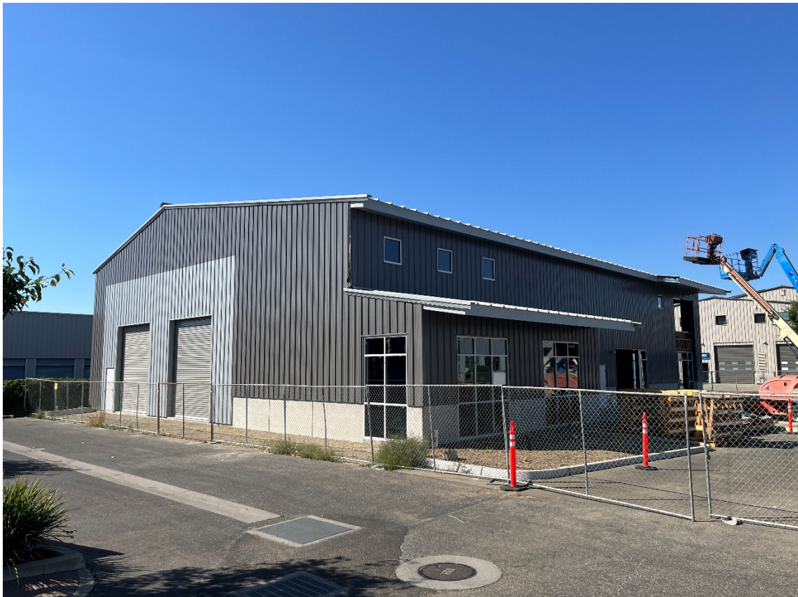
Construction Progress Warehouse Entry
