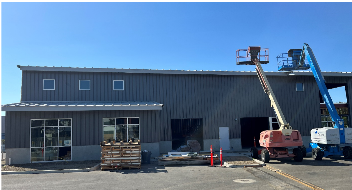
Construction Progress facing Steel Way
