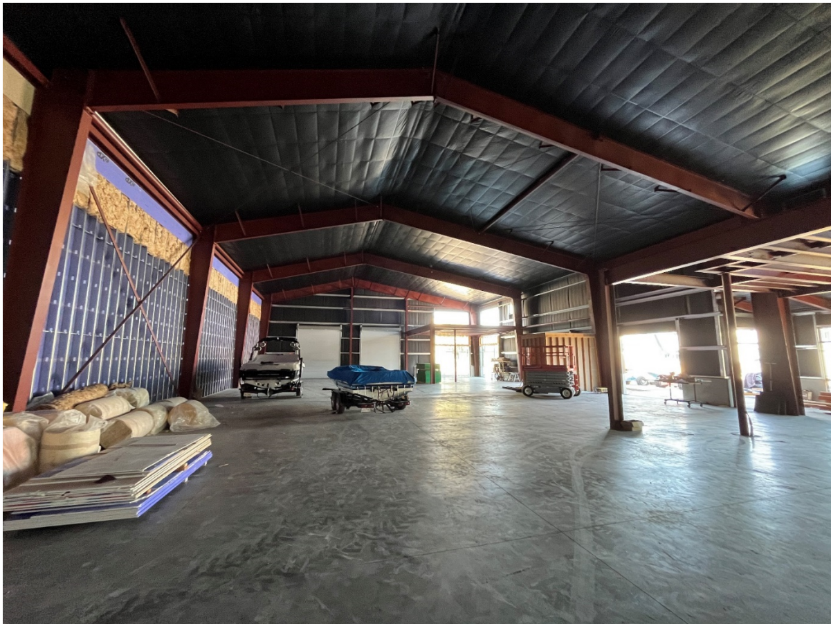
Construction Progress Inside Warehouse
