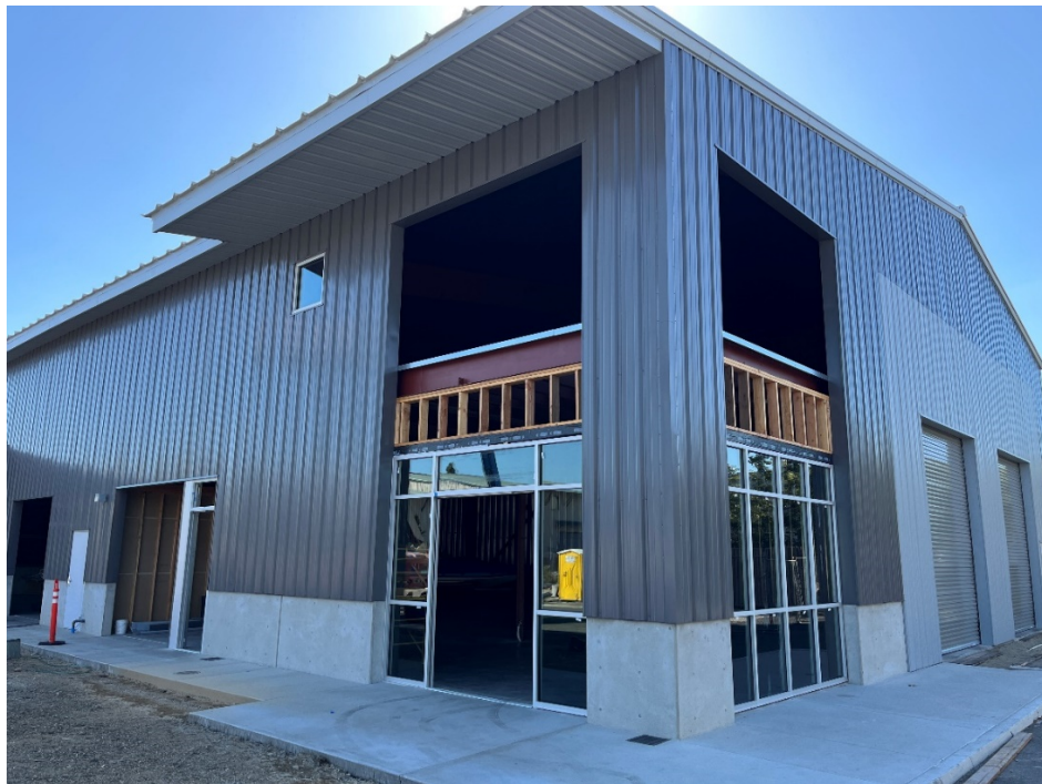
Construction Progress on Main Building Entry
